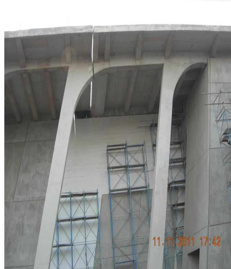
Inclined column and isolated footing with SCC
