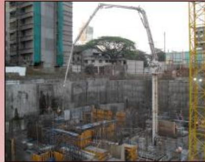
The Orchid Crown project site at Mumbai has achieved the pumping of M-80 grade concrete by pumping it with a BP 2800 concrete pump through 600m concrete pipeline. This is the longest length of pipeline and highest grade of concrete pumped so far among Buildings & Factories sites of L&T. The site has pumped 2500cu.m of M-80 grade concrete so far. Apart from this the site has completed 30,000cu.m of M-60 grade concreting in the last eight months.
